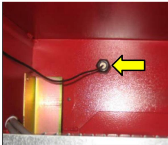
3. Feed the antenna wire through the opening in the back.
