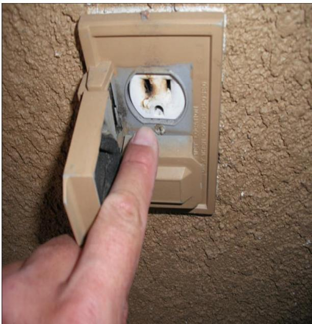
1. Bad Outlet - The actual outlet the GFI is plugged into is bad.
