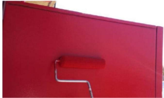
13. Apply second coat. Paint dries quickly in warmer temperatures - approximately10-15 minutes.
