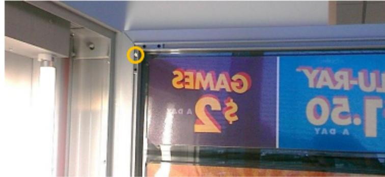
3. Now, remove the side part of the door frame from the light box door. Next, remove the Plexiglass. Careful, as the Plexiglass is not sturdy and will bend and fold over.
